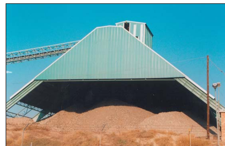
Radon gas emitted from minerals may accumulate in closed storage areas. This can be prevented by storage in well-ventilated sheds
